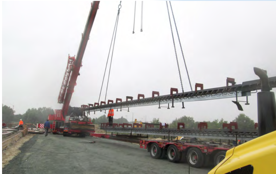
Handling and positioning of multi steel profiles expansion joint
