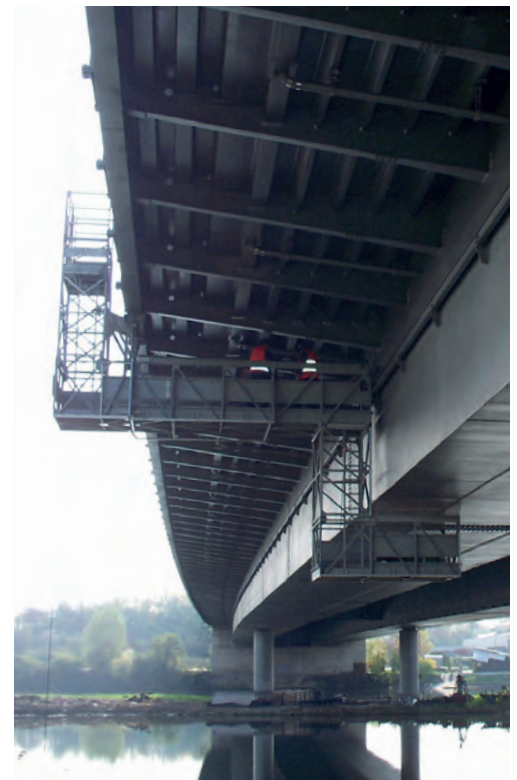
Viaduct over the river Neckar – Germany
