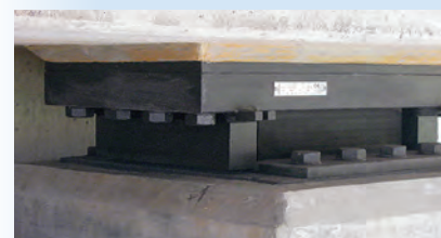
Restrained elastomeric bearing Type VS-RBU installed
