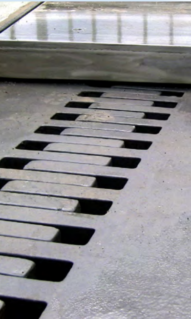
Finger expansion joint with stainless steel sidewalk
