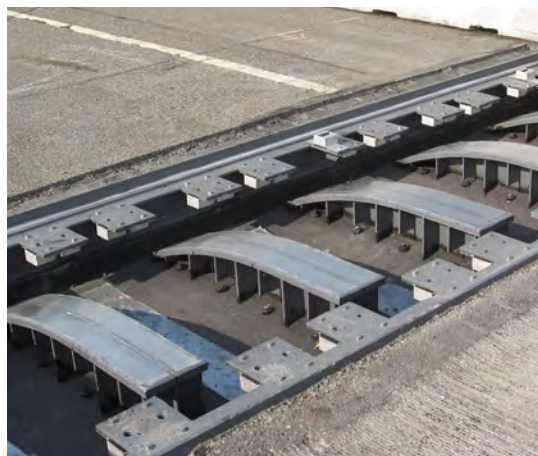
Roller shutter joint during installation
