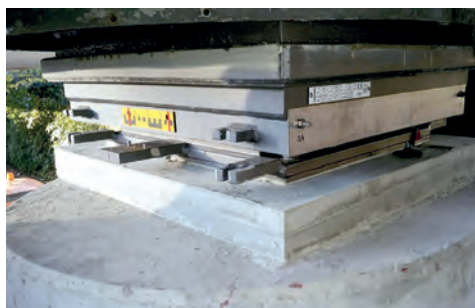
... after installation is completed
