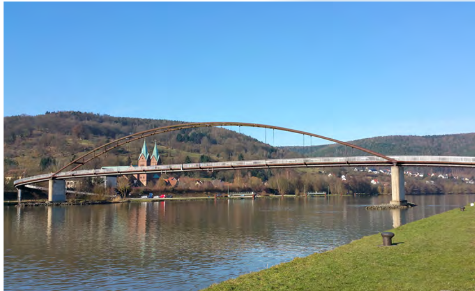
Pedestrian bridge over the river Main – Germany
