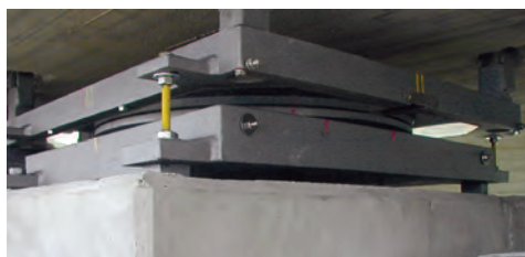
Pot bearings during installation and ...
