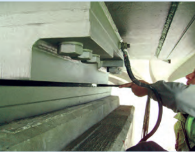
Installation of a fixed shear key
